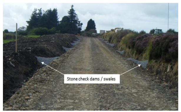
Figure 6-10: Examples of check dams along roadside drainage channels
