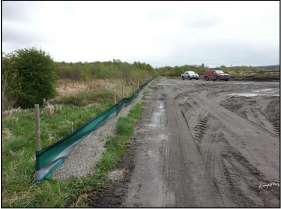
Figure 6-14: Silt curtain containment along existing roads near watercourses
