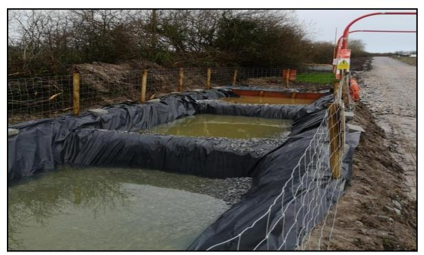
Figure 6-9: Multi-tiered settlement pond with stone filter
