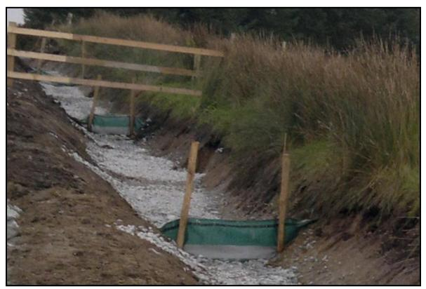
Figure 6-11: Example of a silt fence used in conjunction with check dams along roadside drainage channels
